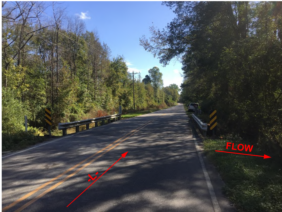
Photograph No. 2: View of -L- and Big Shoe Heel Creek looking east.
